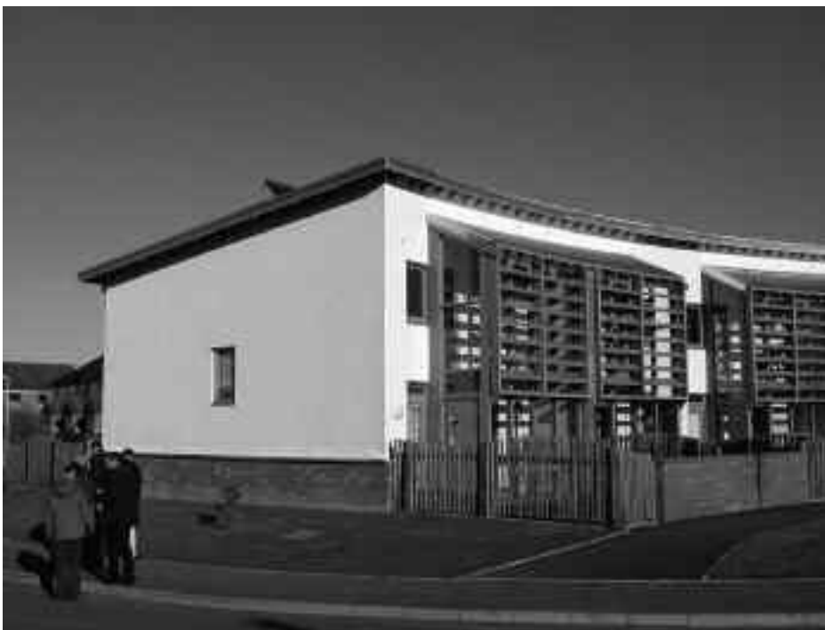
Low energy housing by South Shropshire Housing Association, Craven Arms
